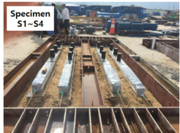
Fig. 5 Steel test frame and the specimens(S1~S4)
