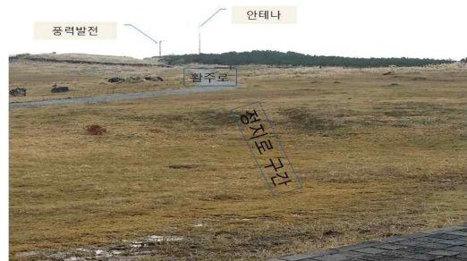
Fig. 3 Predicted slope emergency runway of Marado
