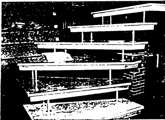
Fig.7 Staircase units without walls
