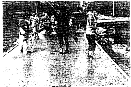
Fig. 3. Casting Recycled Concrete by Hand in the Field
