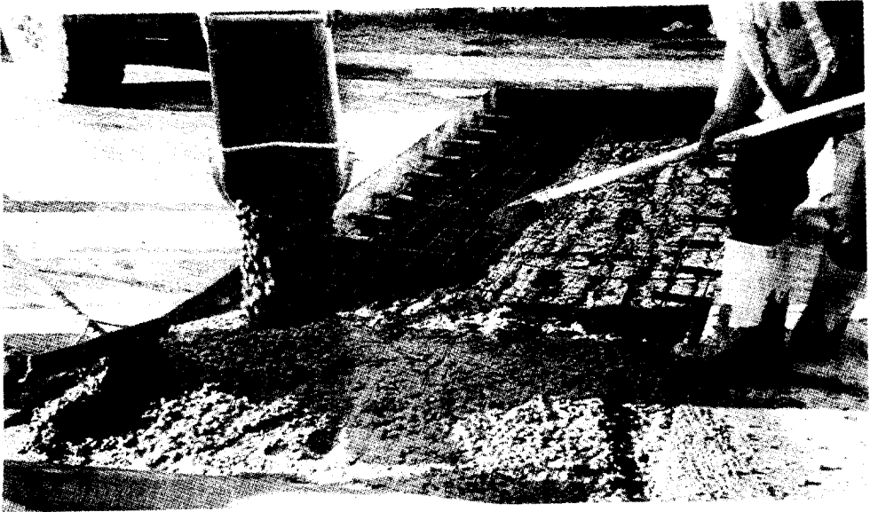
Figure 18. Placement of Concrete in the Patch.
