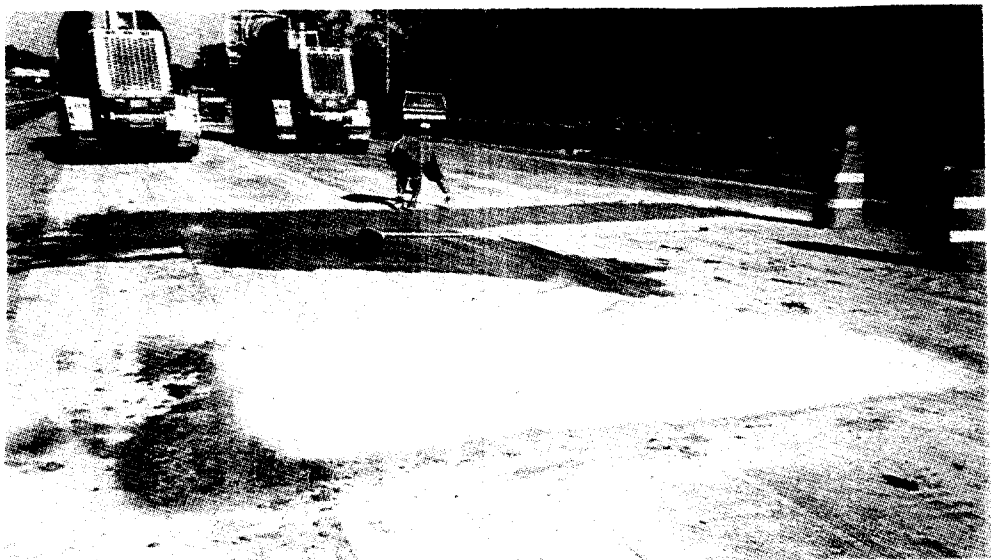
Figure 19. A Completed Patch.
