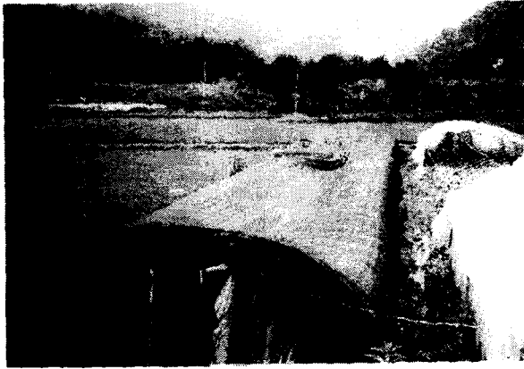
Fig. 1. Deformed shape of Shiitake cultivation facilities.
