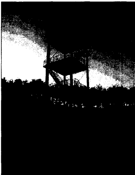
Fig. 1 Test Structure(Unison Tower)
