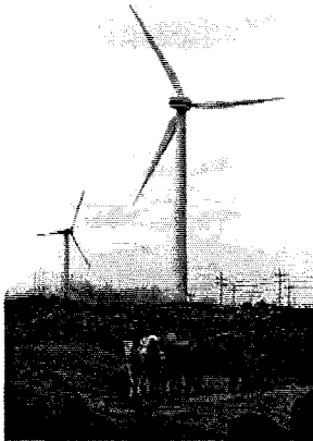
<Fig. 3> Hangwon wind farm
