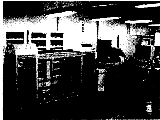
Fig. 11 Automatic Function Test System
