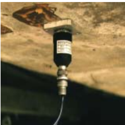
Fig.5 Accelerometer attached on the tank
