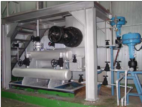
Fig. 13 steam & high press. gas test line
