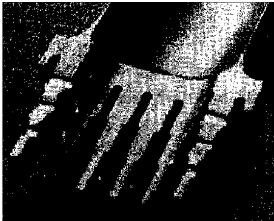
Fig. 4 Pinned finger dovetail
