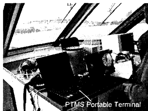
Fig.4 PTMS portable terminal installed on the bridge of "Ootaka"
