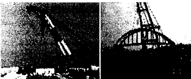
Photo 6 a view of Caisson deposition and on the sea bridge installation
