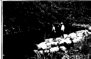
Photo 5. Concrete Deflector with Rock Coating
