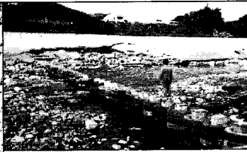
Photo 3. Tire weir with opening
