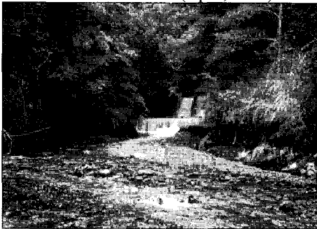
Photo 3. Dam No.3 (October, 1997)
