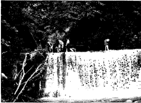
Photo 1. Dam No.4 (April, 1999)
