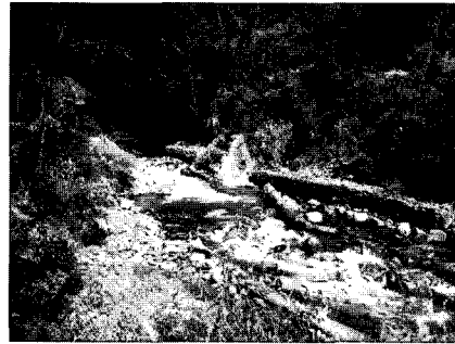
Photo 2. Dam No.4 (October, 2001)
