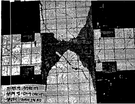
Fig. 10 Failure of PBC 2
