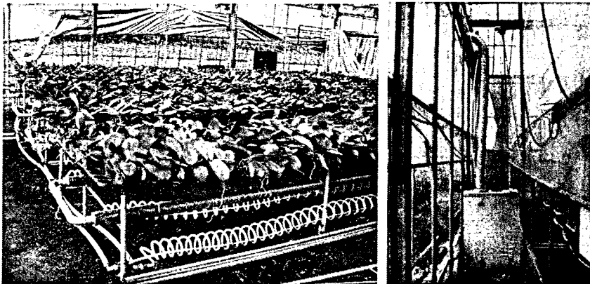
Fig. 10. Coil tube heat exchange system installed in Phalaenopsis cultivation greenhouse.
