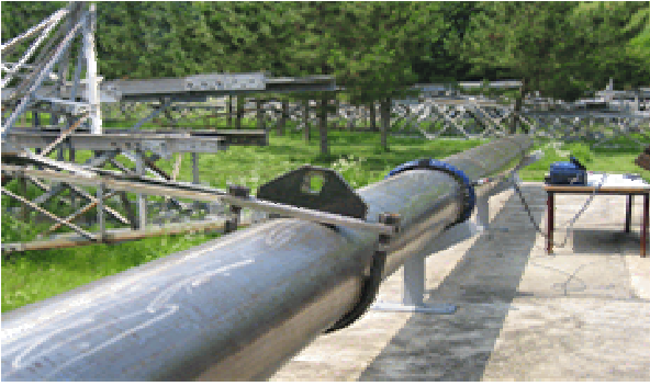
Fig. 3 Photo of the large-diameter pipe
