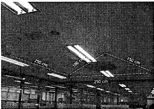
Fig. 2. Deployment of the Beacons in the Ceilings for Test.
