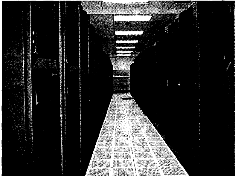
Figure 1. Photograph of data center computer equipment
