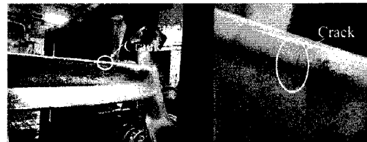
Fig. 4 Crack resulted from the durability test
