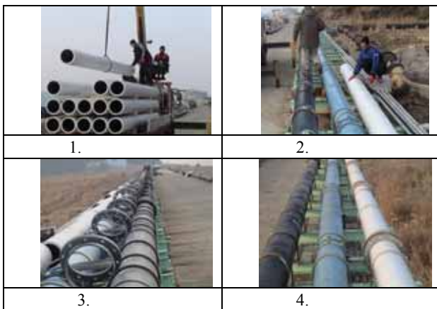
Fig. 4 . Installation of prototype FRP pipe
