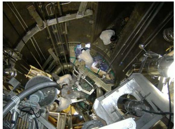
Fig 7 Installation of In-Pile Section
