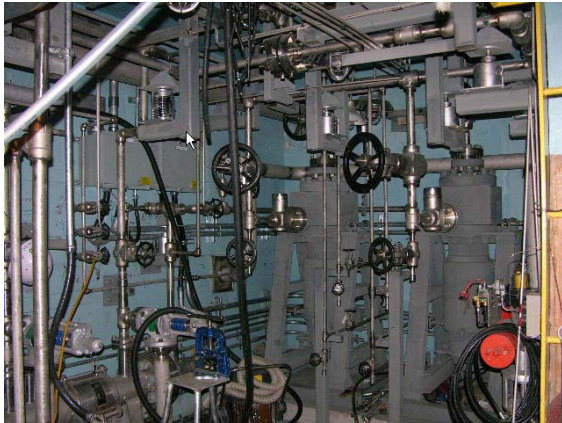
Fig. 5 Construction of Room #1
