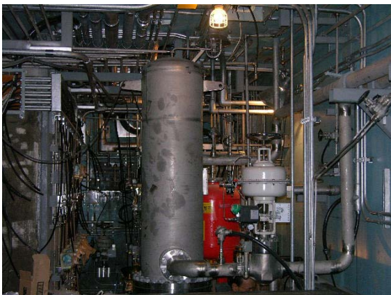
Fig. 6 Construction of Room #2
