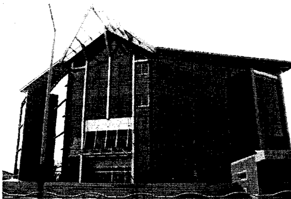
Picture. 1 The Building for Extruding ground water source heat pump operation.
