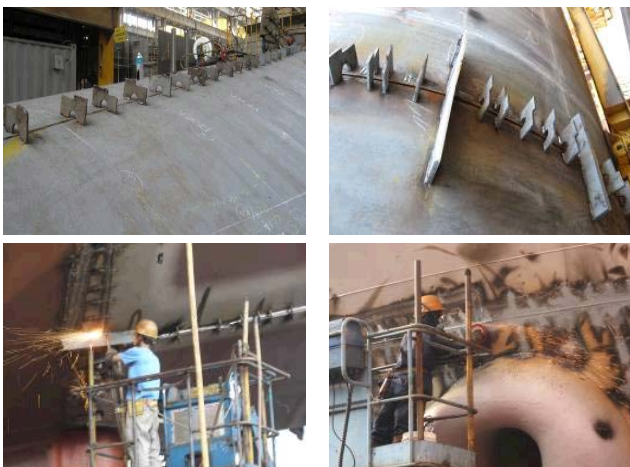
Fig. 1 Removing work of Bead and Piece
