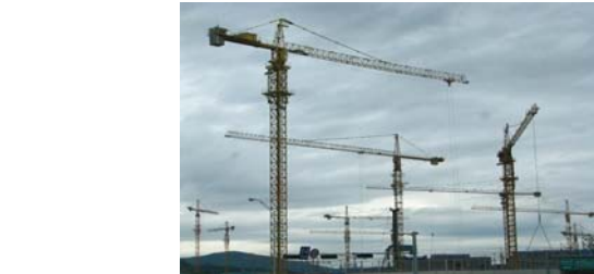
Fig. 1 Tower crane at the construction site
