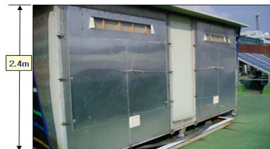
Figure 2. KIER twin test cell.
