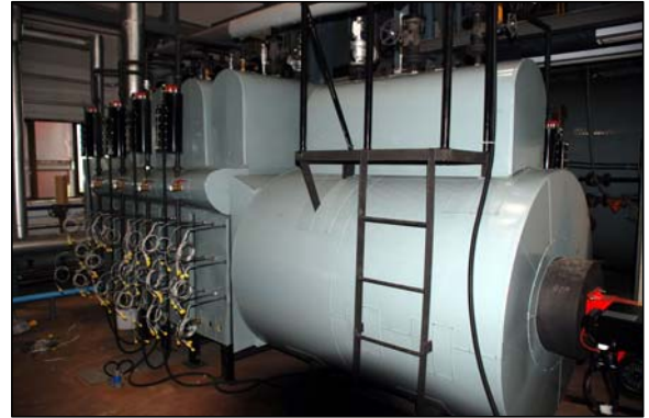
Fig. 2 Installation of boiler and heat exchanger.
