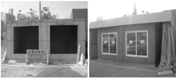
Fig. 4 Installation of protection tent
