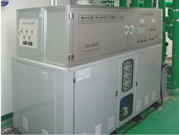
Fig. 3 Heat pump system
