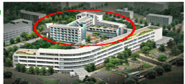
Fig. 1 Building of the ground source heat pump installed.
