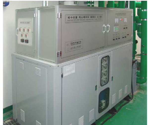
Fig. 2 Sea water source heat pump system
