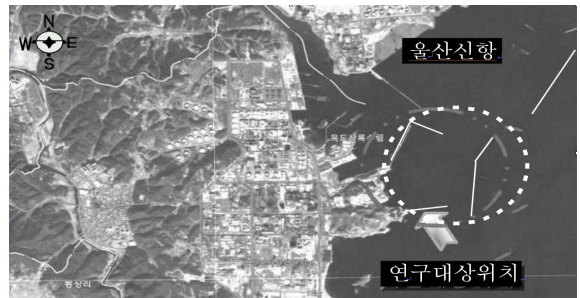
Fig. 1. Location of Ulsan south breakwater
