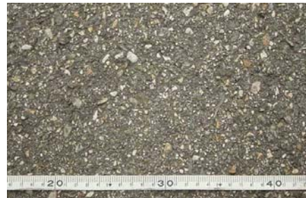
Fig.3 The test road
