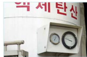
Fig. 1 Analog type measuring device of a gas level
