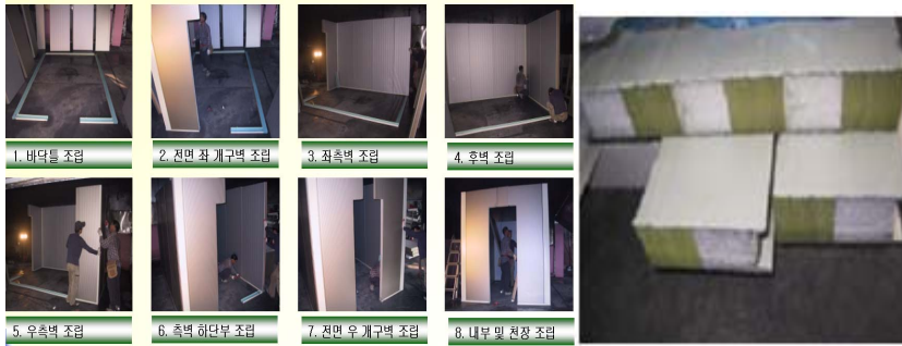
Figure 1 Assembling Process and Specimen material
