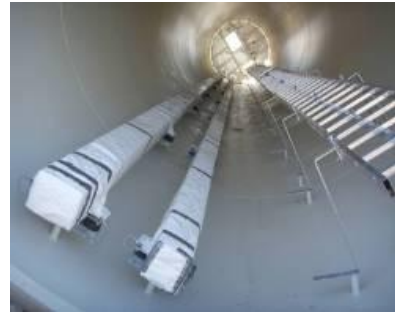
Fig. 6 Bus Trunk Installation on Tower Section
