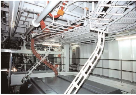
(a) Cable Installation
