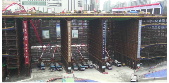
Figure 6. Underground Placement of Pump-car
