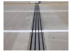
(c) Rail joint
