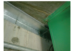
(c) After installation
