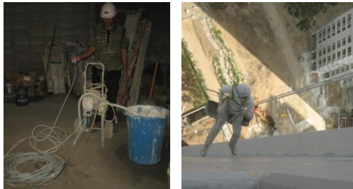
Fig. 1 Conventional painting work and tools
