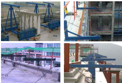
Fig. 1 Temporary gondola supporting means
