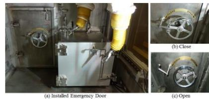
Fig. 4. Emergency door operated by MSM.
