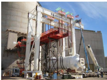
Fig. 1. Example of Steam Generator Withdrawal in ZORITA NPP.
