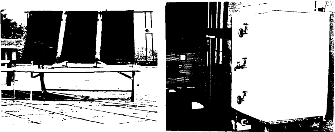
Fig.2 Photo of Solar Water Heating Systems.
