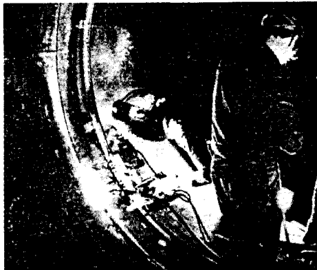
Weld position, vertical up
