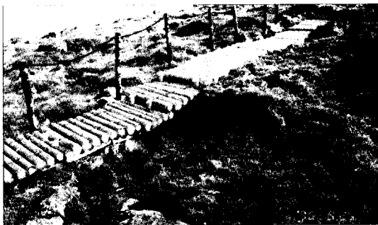
Photo 10-1. Current view of long-walkway
