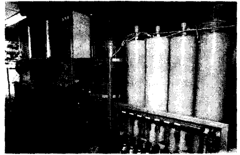
Fig. 1. Photograph of the pilot plant.
