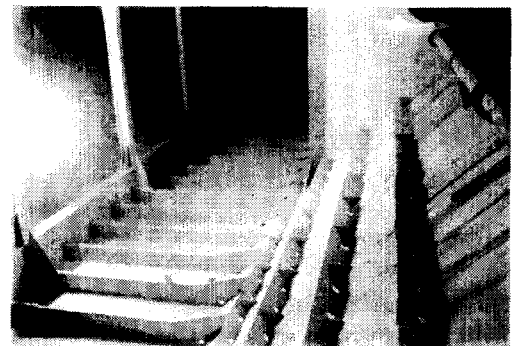
Photo. 10 Protection for fresh water tank inside
