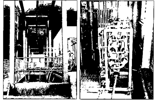
Fig 3. Photograph of yongin-gun leachate treatment facility
